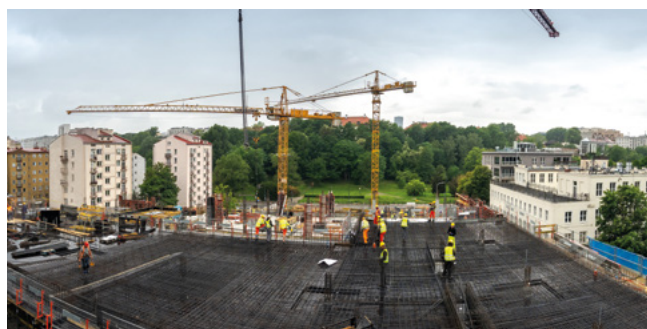
v The construction work at Dobra 55 (the second stage).
